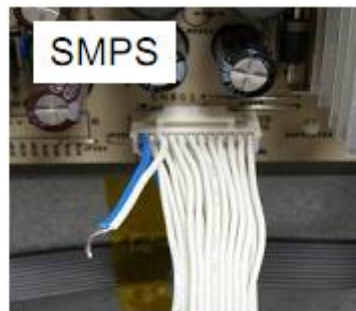
Short the PS_ON and GND pins on the ribbon cable connector from Main Board to SMPS (24P)
